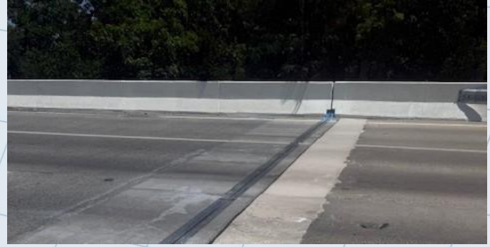
View of approach slab on a recently treated bridge that applied a rapid curing concrete
