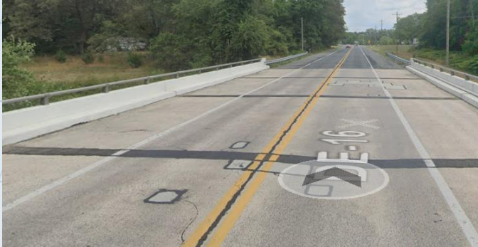
View of deck on a recently treated bridge with repaired patches and hot poured joint sealer to protect from further water intrusion
